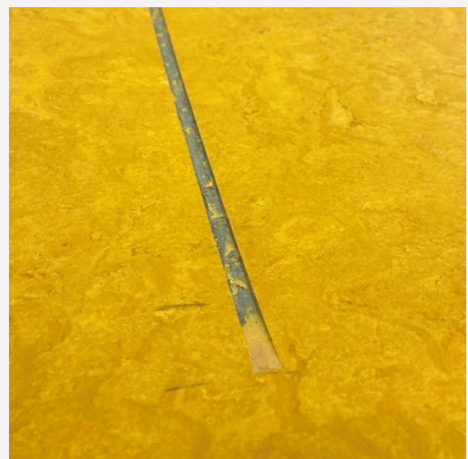
Cutting 'ramps' on either end of all rebates.
